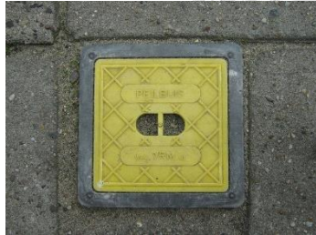
Connected measuring tube groundwater level
